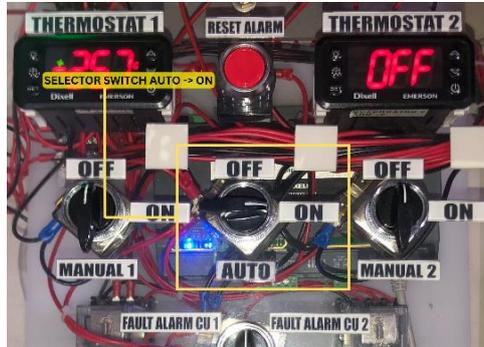
Gambar 12. Kondisi *Selector Switch* saat Mode Auto
