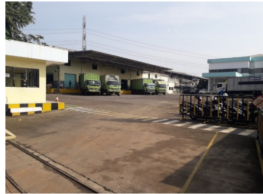
Gambar 1. Area Loading Warehouse Finish good PT. SGB
